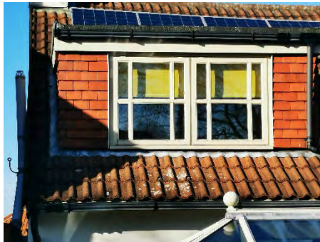
View of timber window to rear dormer.
