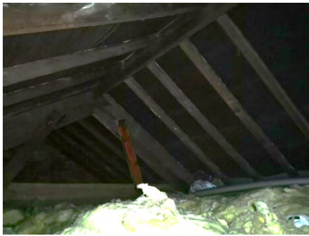
View of secondary roof sub-structure.
