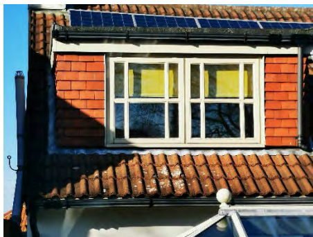
View of fascia to rear dormer.
