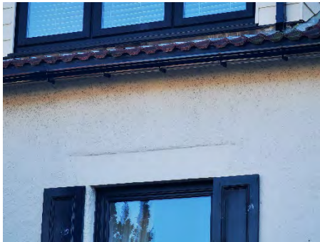
View of guttering to front roof pitch.
