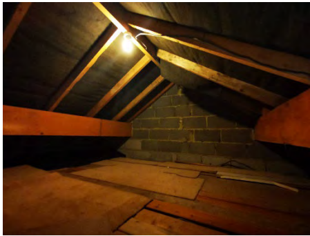
View of secondary roof sub-structure.
