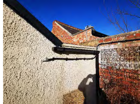
View of guttering to rear extension flat roof.
