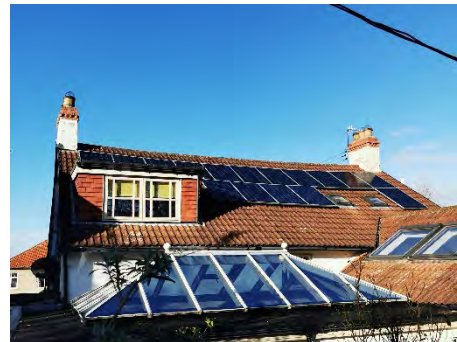
View of rear roof pitch.
