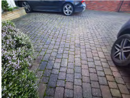
View of driveway covering.
