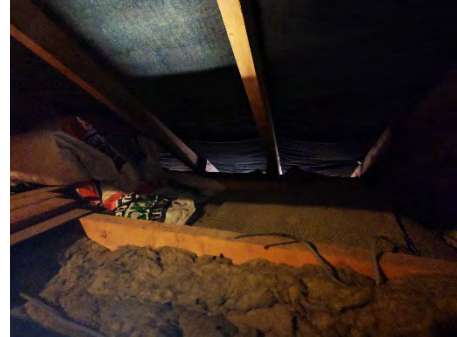
View of underlay to secondary roof.
