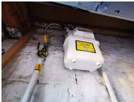
View of gas supply location.
