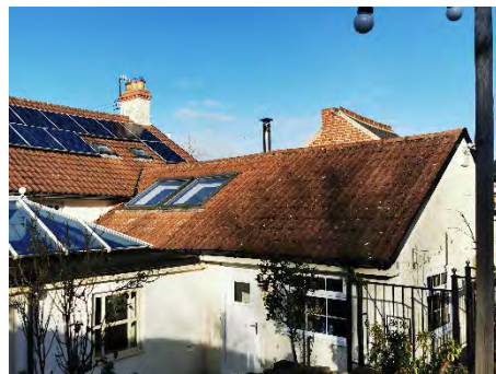
View of pitched roof to rear extension.
