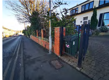
View of front boundary wall.
