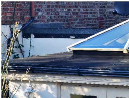
View of flat roof serving kitchen.
