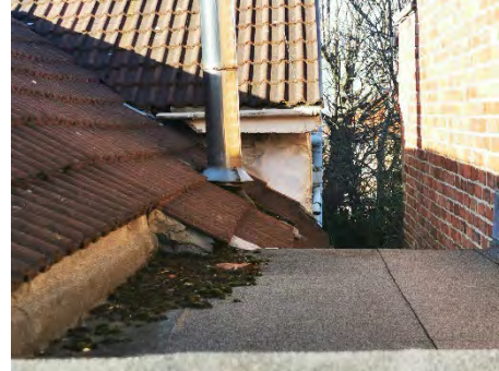
View of flue to rear dining room fireplace.
