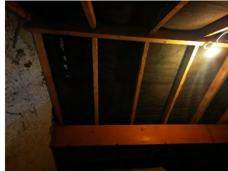
View of secondary roof sub-structure.
