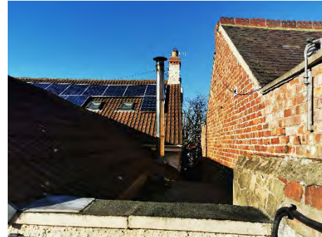
View of flat roof to rear extension.
