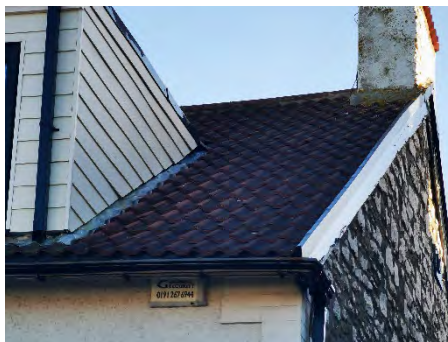
View of front roof pitch.
