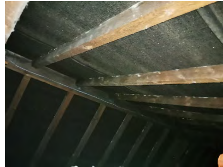
View of secondary roof sub-structure.
