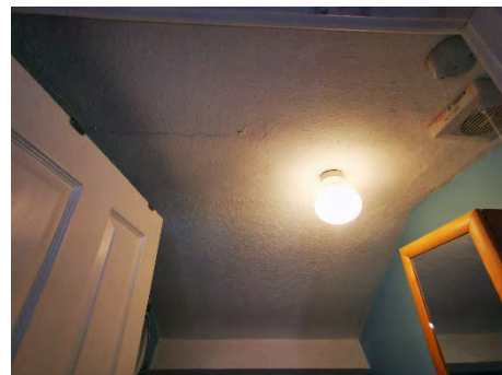
View of en-suite bathroom.
