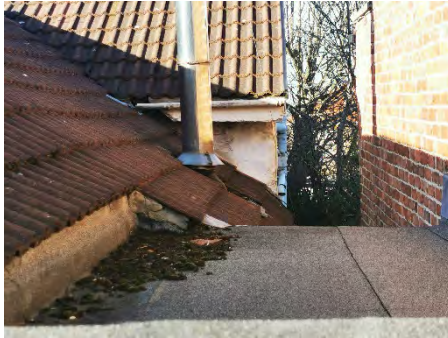
View of flat roof to rear extension.
