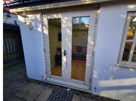
View of rear double leaf door serving kitchen extension.
