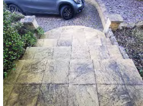
View of steps to front entrance.
