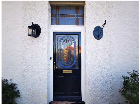
View of front entrance door.
