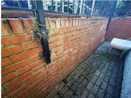
View of rear retaining wall.
