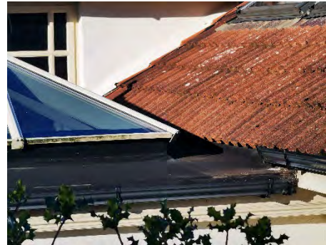
View of flat roof serving kitchen.
