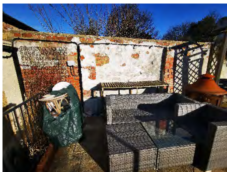
View of rear wall.
