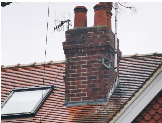
3. Front chimney serving front reception room.
