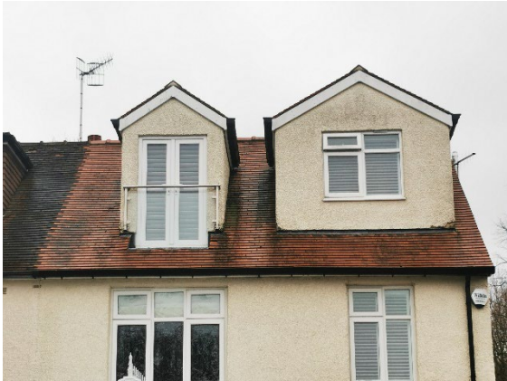
13. Rear roof pitch.
