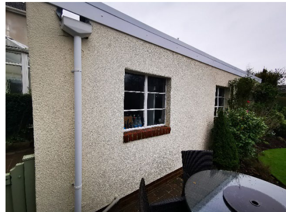
16. Side elevation to garage.
