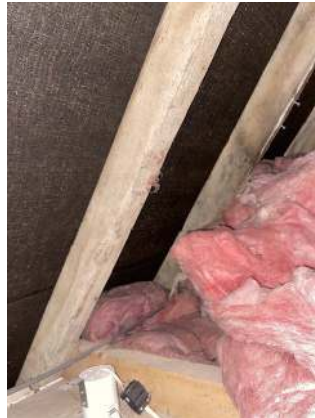
Second floor bedroom roof void
