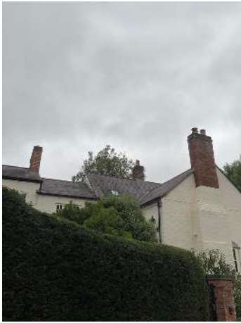
15. View of chimney stacks
