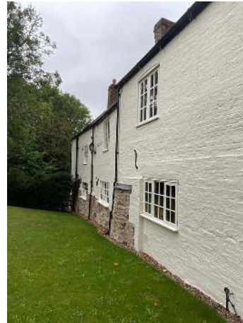
28. Rear elevation windows
