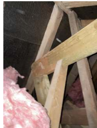
Second floor bedroom roof void
