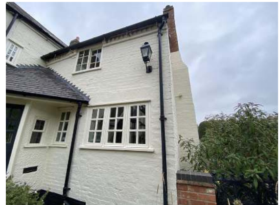
Timber fascias and brick gutter shelf
