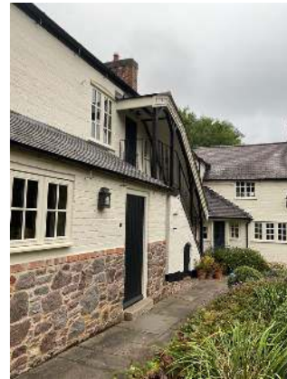
Front elevation rainwater goods
