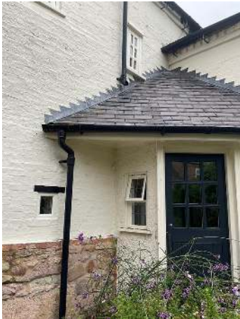
33. Timber fascias and brick gutter shelf
