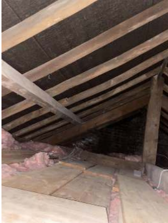
61. Main roof void accessed via first floor landing
