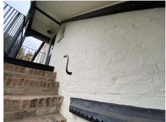
Wall plate installation
