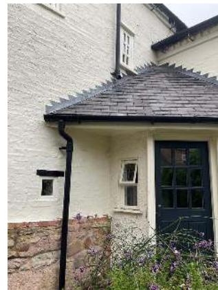
Timber fascias and brick gutter shelf
