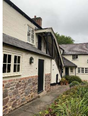
20. Front elevation rainwater goods
