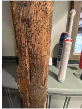
Evidence of wood boring beetle within first floor bathroom
