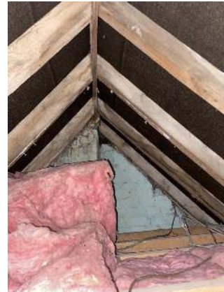
Second floor bedroom roof void
