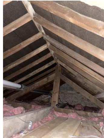
64. Main roof void accessed via first floor landing
