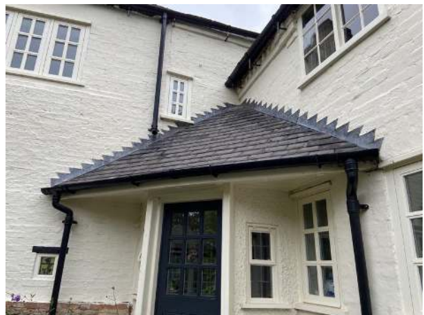
12. Side porch roof covering
