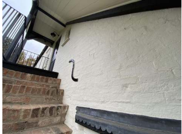
8. Wall plate installation
