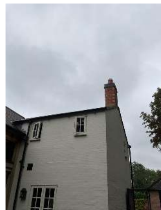
Rear view of chimneys
