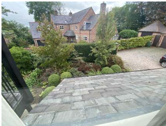
Front porch roof covering
