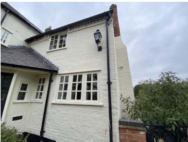
35. Timber fascias and brick gutter shelf
