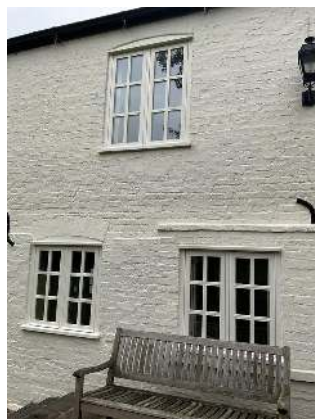
Rear elevation windows
