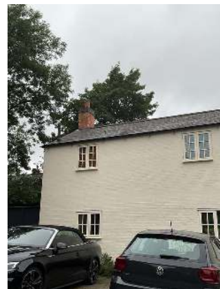
View of chimney stack
