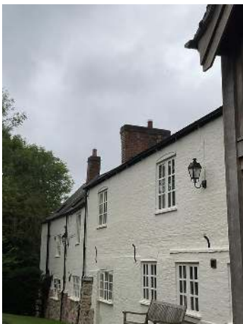
17. View of rear chimneys
