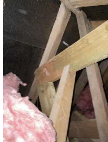
68. Second floor bedroom roof void
