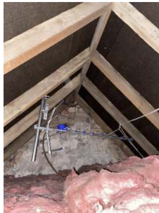
Second floor bedroom roof void
