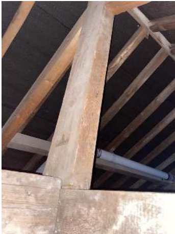
63. Main roof void accessed via first floor landing
