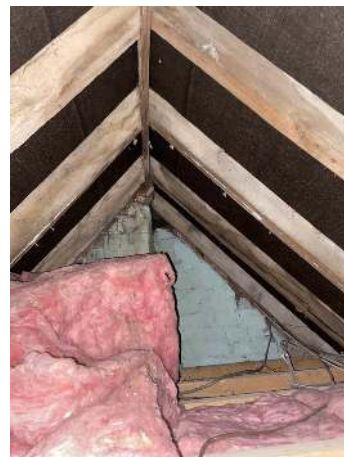
66. Second floor bedroom roof void
