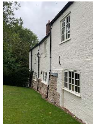
Rear elevation rainwater goods
