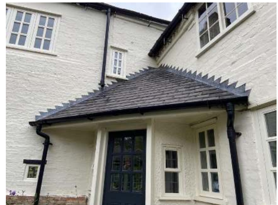
Side porch roof covering
