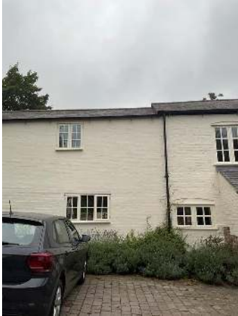
19. Front elevation rainwater goods
