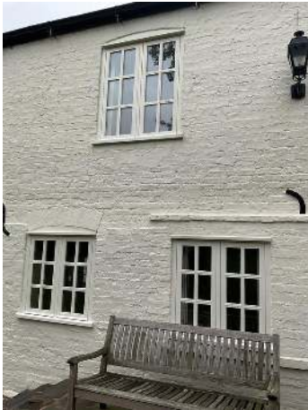
27. Rear elevation windows
