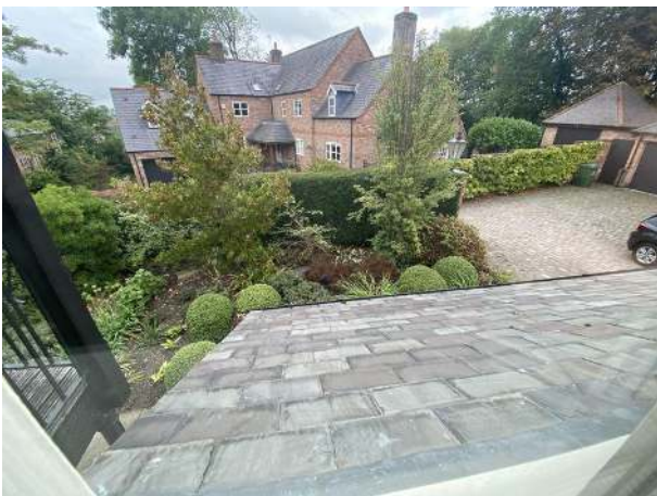
11. Front porch roof covering
