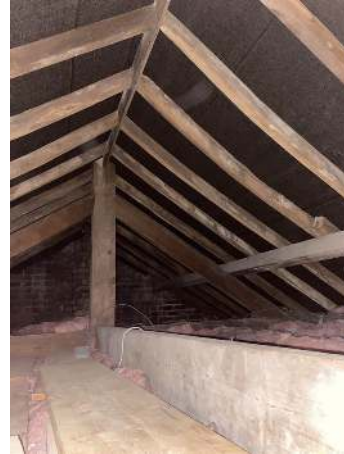
62. Main roof void accessed via first floor landing
