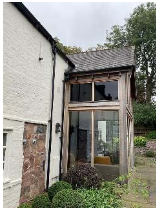
Rear elevation rainwater goods
