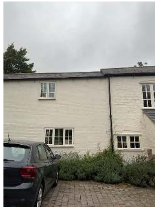
Front elevation rainwater goods
