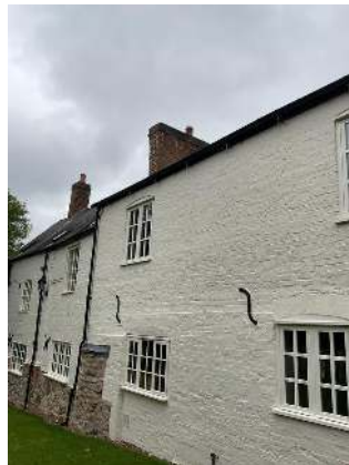
Rear elevation external joinery
