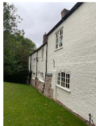
Rear elevation windows
