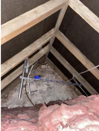
67. Second floor bedroom roof void
