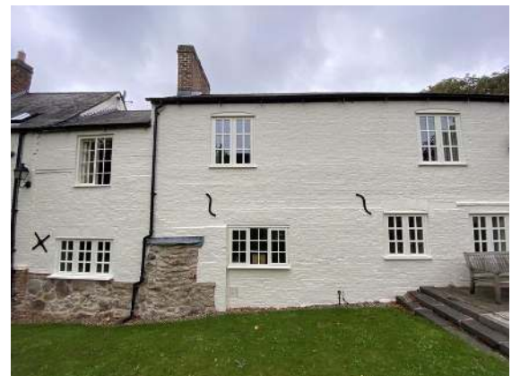
Wall plate installation
