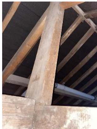
Main roof void accessed via first floor landing
