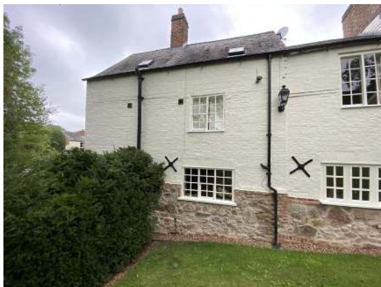
Wall plate installation
