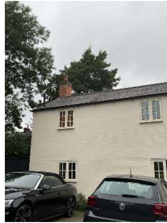
16. View of chimney stack
