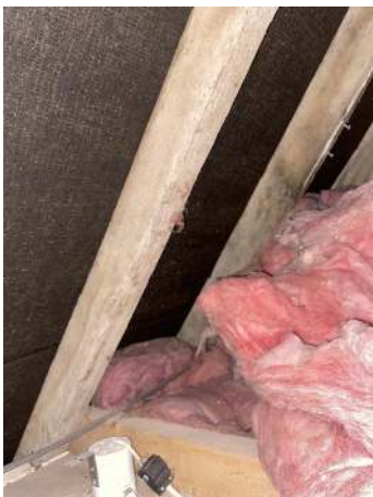
65. Second floor bedroom roof void
