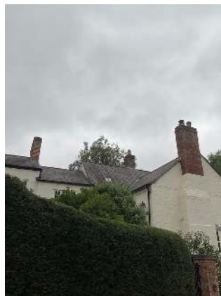
View of chimney stacks
