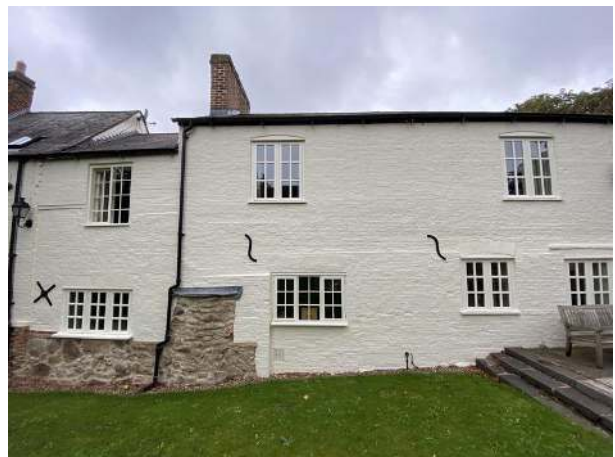
6. Wall plate installation
