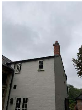
18. Rear view of chimneys
