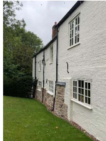
22. Rear elevation rainwater goods
