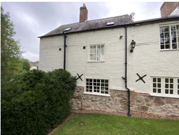
5. Wall plate installation
