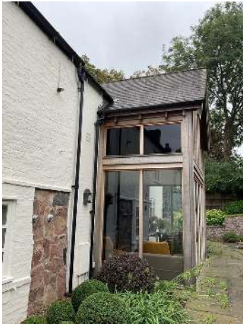
21. Rear elevation rainwater goods
