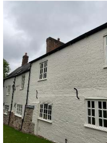
34. Rear elevation external joinery
