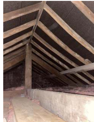
Main roof void accessed via first floor landing
