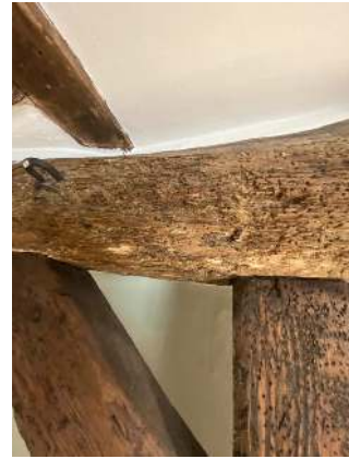
Evidence of wood boring beetle within first floor bathroom
