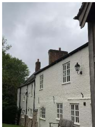
View of rear chimneys
