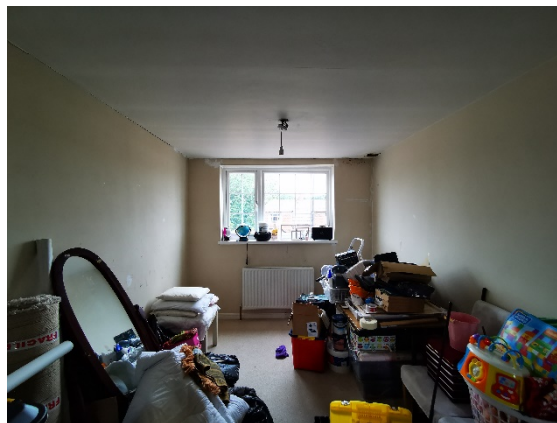
View of plasterwork to first floor.
