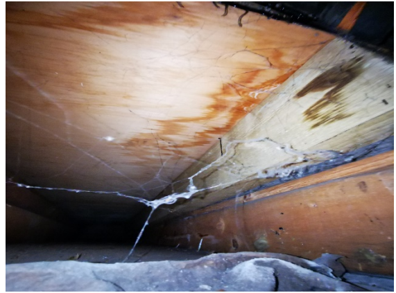
View of flat roof void.
