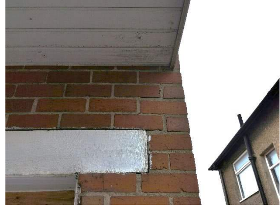
View of brickwork to front elevation garage lintel.
