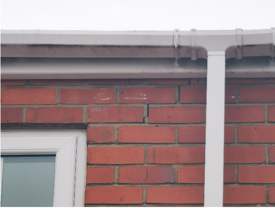
Brickwork to front elevation first floor window.
