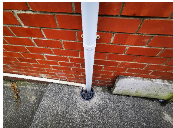
View of drainage inlet to side elevation.
