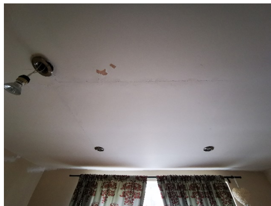
View of plasterwork to first floor.
